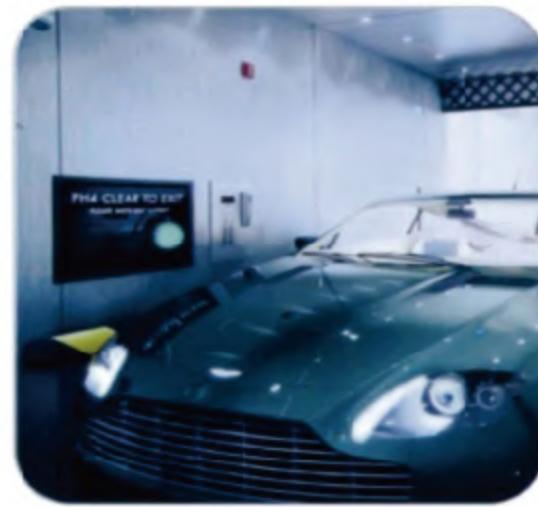
⚡ Special-purpose circuit control and display system
